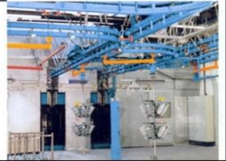
Blast cleaning of aluminum parts on a Power and Free system
